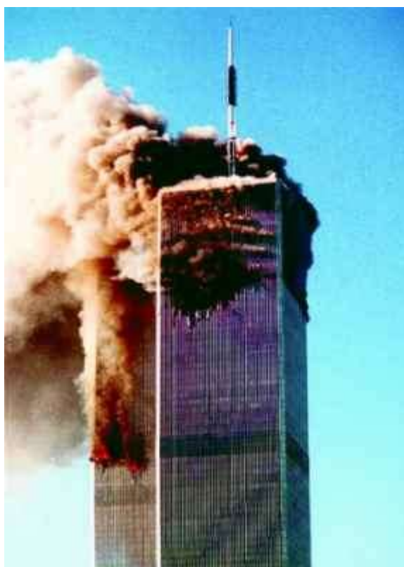
Figure 2-30 North face of WTC 2 opposite the zone of impact on the south face, behind WTC 1.
