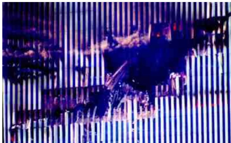
Figure 2-15 Impact damage to the north face of WTC 1.
