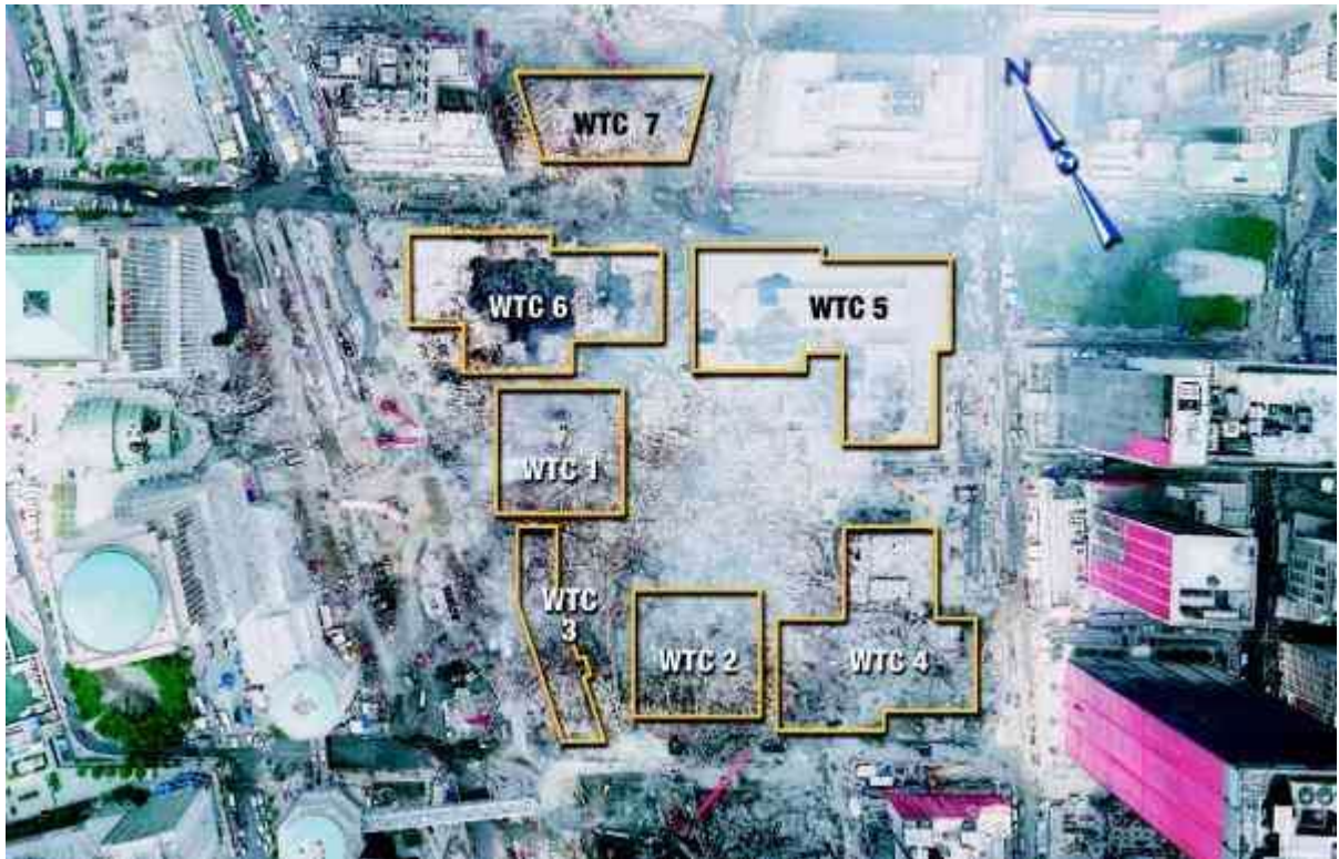
Figure 2-23 Aerial photograph of the WTC site after September 11 attack showing adjacent buildings damaged by debris from the collapse of WTC 1.
