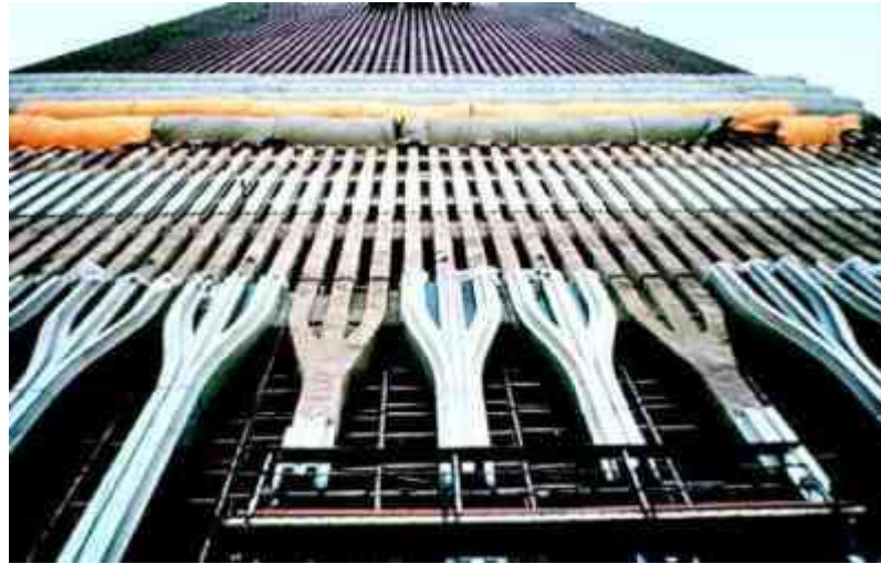
Figure 2-4 Base of exterior wall frame.
