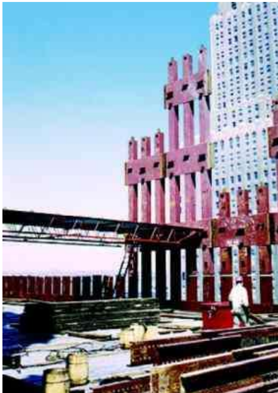
Figure 2-8 Shows the erection of floor framing during original construction.
