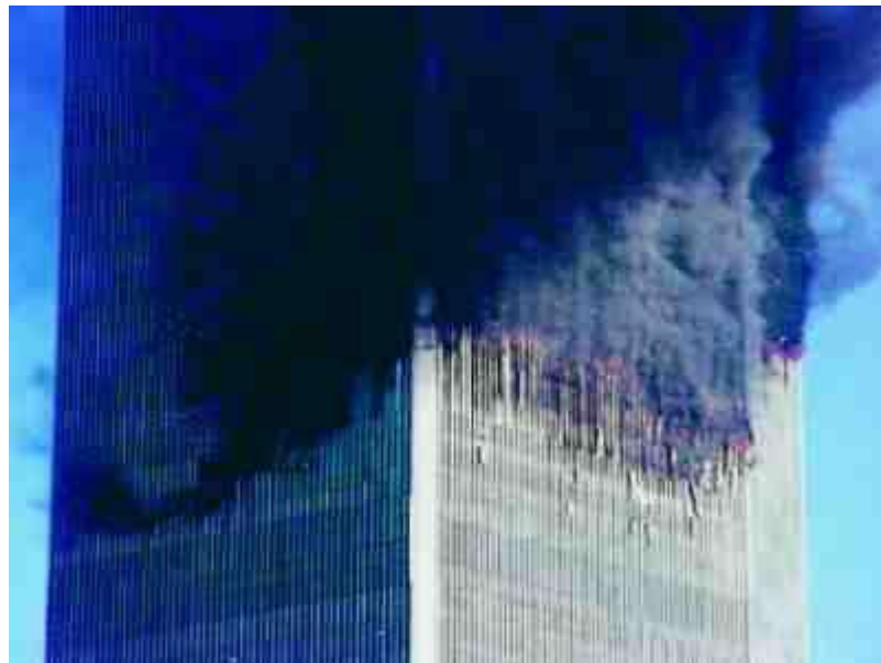
Figure 2-26 Impact damage to the south and east faces of WTC 2.
