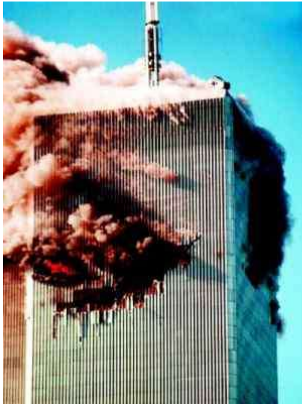
Figure 2-13 Zone of aircraft impact on the north face of WTC 1.
