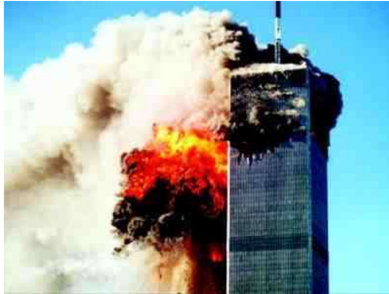
Figure 2-28 Conflagration and debris exiting the north wall of WTC 2, behind WTC 1.
